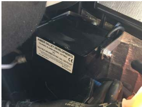
Images 4.2 – Siren screwed firmly into place
