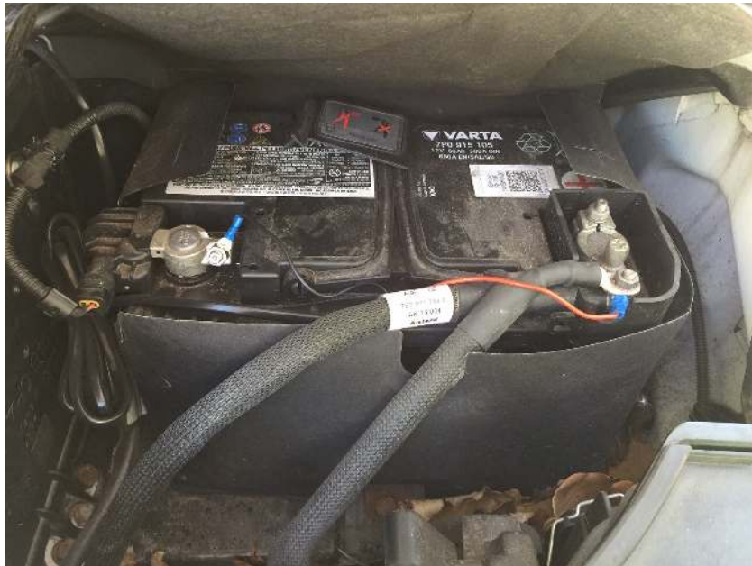
Images 5.1 – Battery connection
